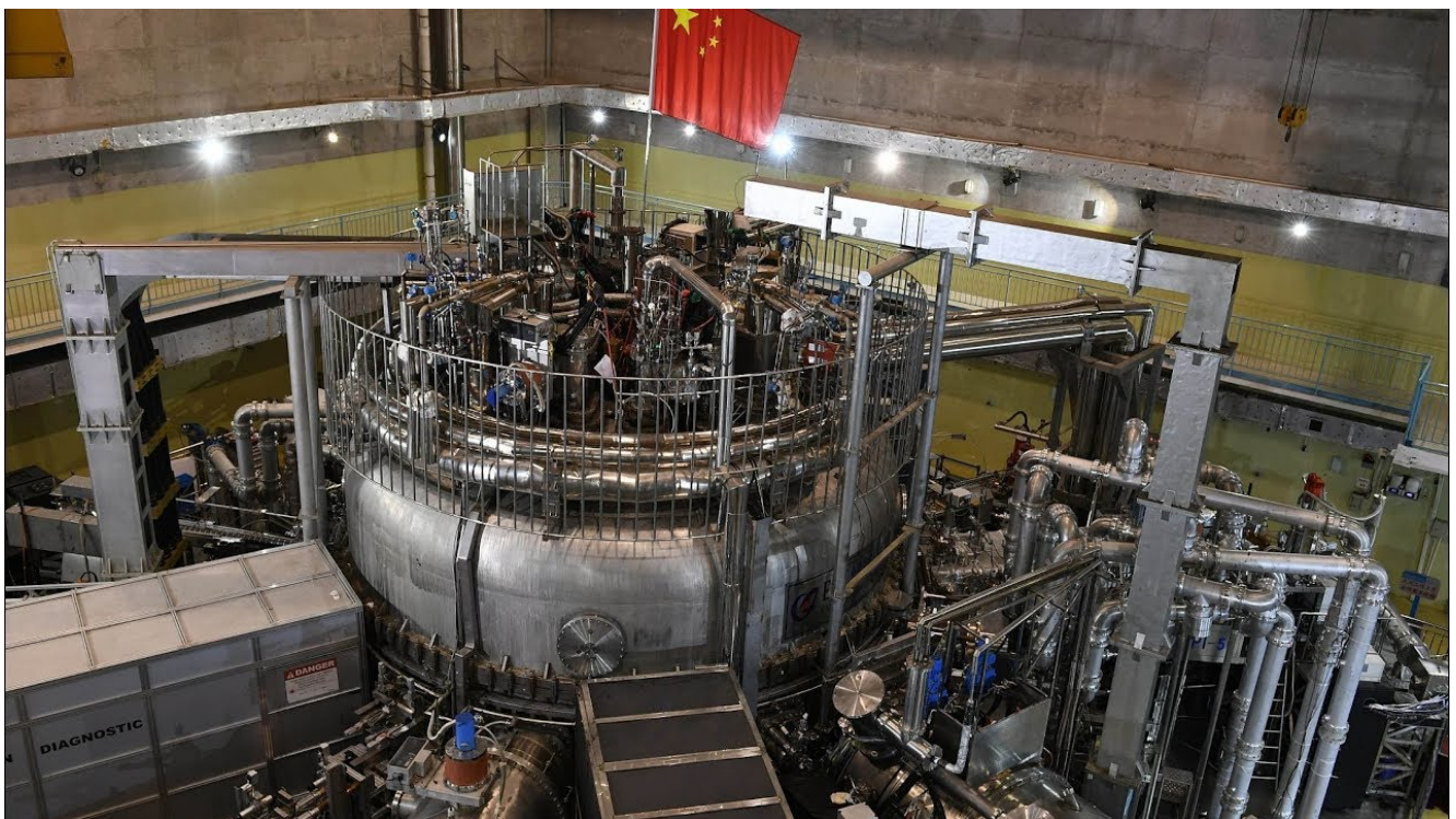
Construction of China's EAST Tokamak reactor within the site [Image Credits: Chinese Academy of Sciences]
